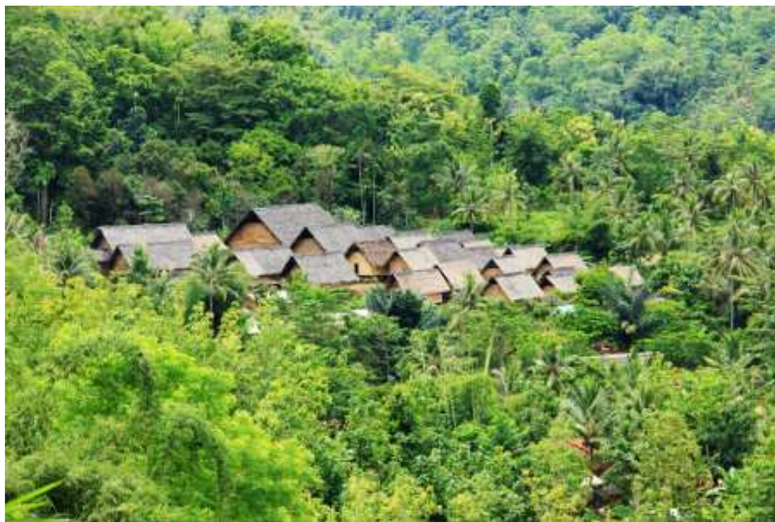
Figure 1. A picture of the Dukuh Traditional Village with its simple and distinctive houses. [Source: indonesiakaya.com ]
