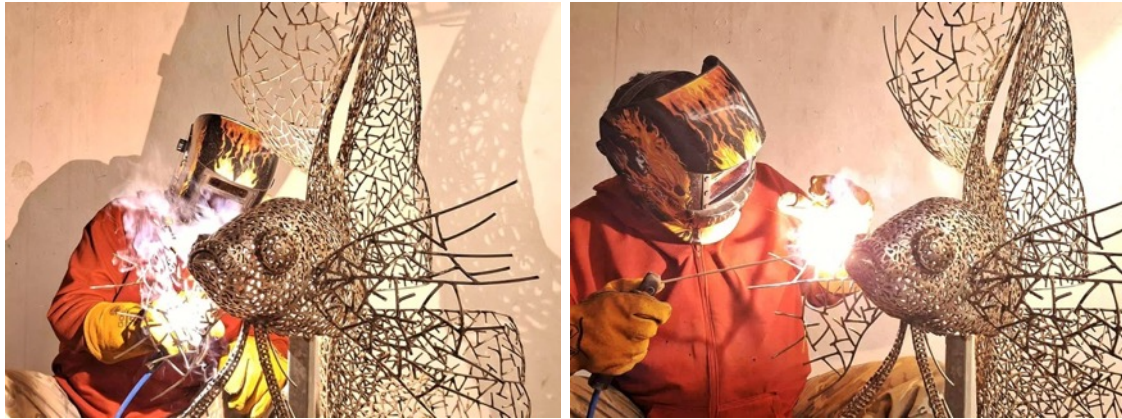
Figure 8. Perpendicular Welding Position to The Welding Object (Left). Angled Welding Position Leaning to The Right of The Welding Object (Right). [Source: Research Team, 2025]
